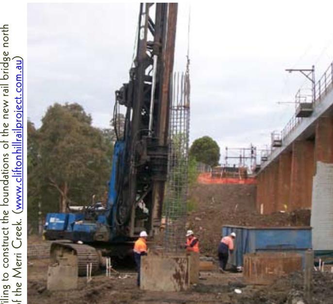
Piling to construct the foundations of the new rail bridge north of the Merri Creek. ([www.cliftonhillrailproject.com.au](http://www.cliftonhillrailproject.com.au))
